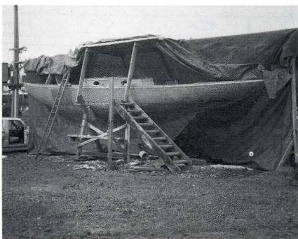
Work in progress: the doghouse removed and the paint stripped. (McGlashan collection)
